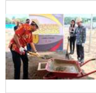
Ground breaking of FKT new LOBP in Cilegon, Banten
